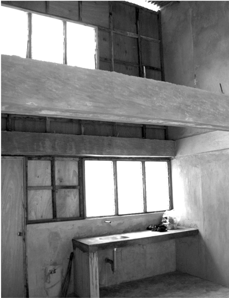
Housing unit in shell condition. In this condition, a housing unit is handed over to the new homepartners and their families.
